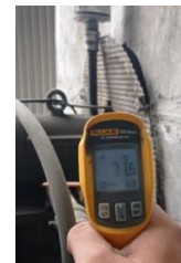
Gambar 6. Temperature Bearing Fan 482-FN5 Free Side setelah instalasi
